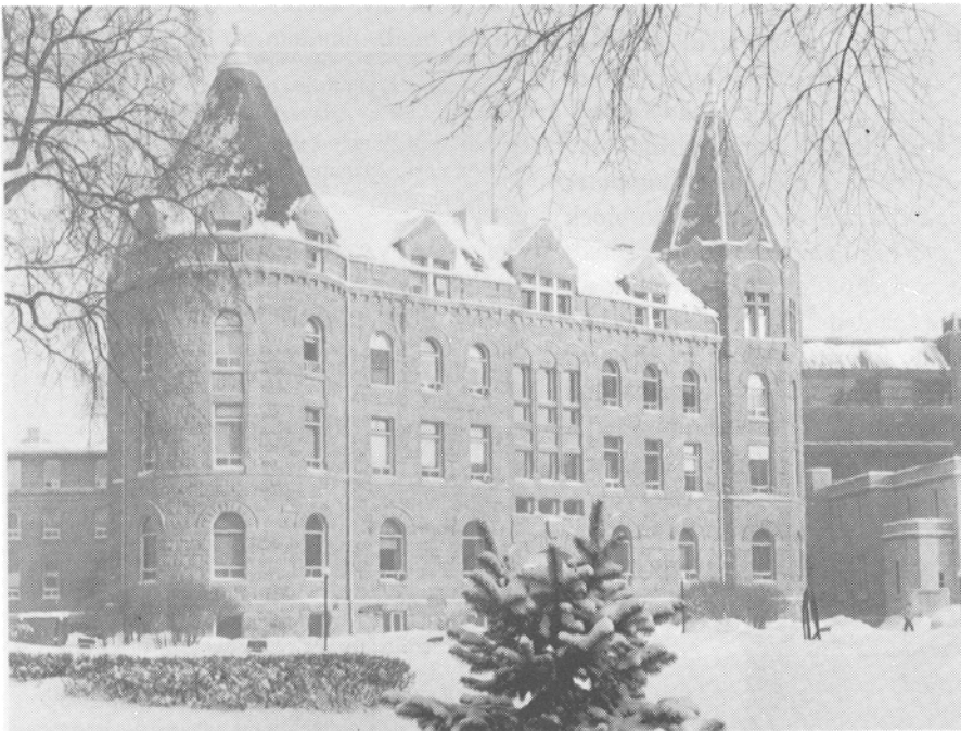
When a dramatic acceleration of structural movement in Wesley Hall became apparent, staff were quickly relocated out of the affected area.
